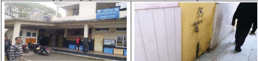
TCC building, Nalbari is used by Addl. CM&HO. Equipment were kept in locked room (photograph taken on 24 & 27 January 2020)
